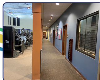
Fitness Center Hallway – Before
