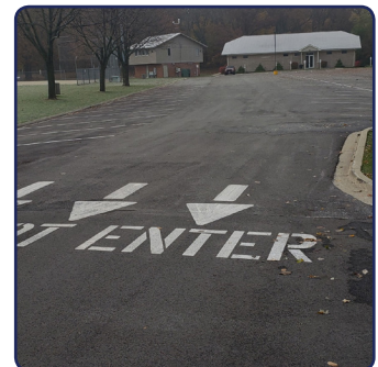
Main Park Parking Lot Resurfacing
