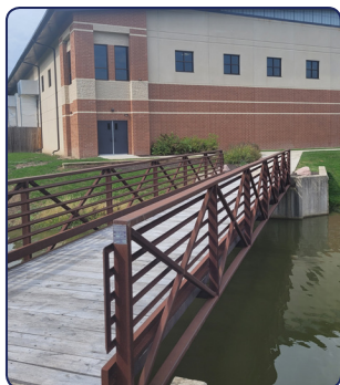
New Deck on the Oaks Disc Golf Course Bridge
